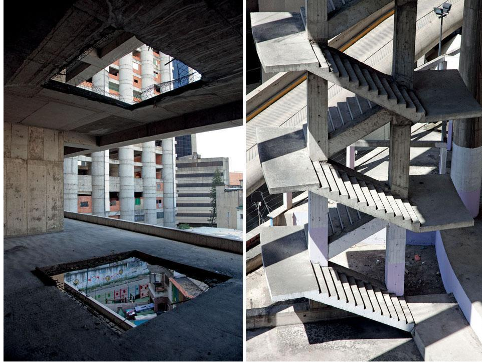
Figure 28. Vertical Cores in the Tower of David
