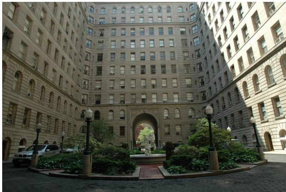
Figure 41. View of the Apthorp Courtyard
