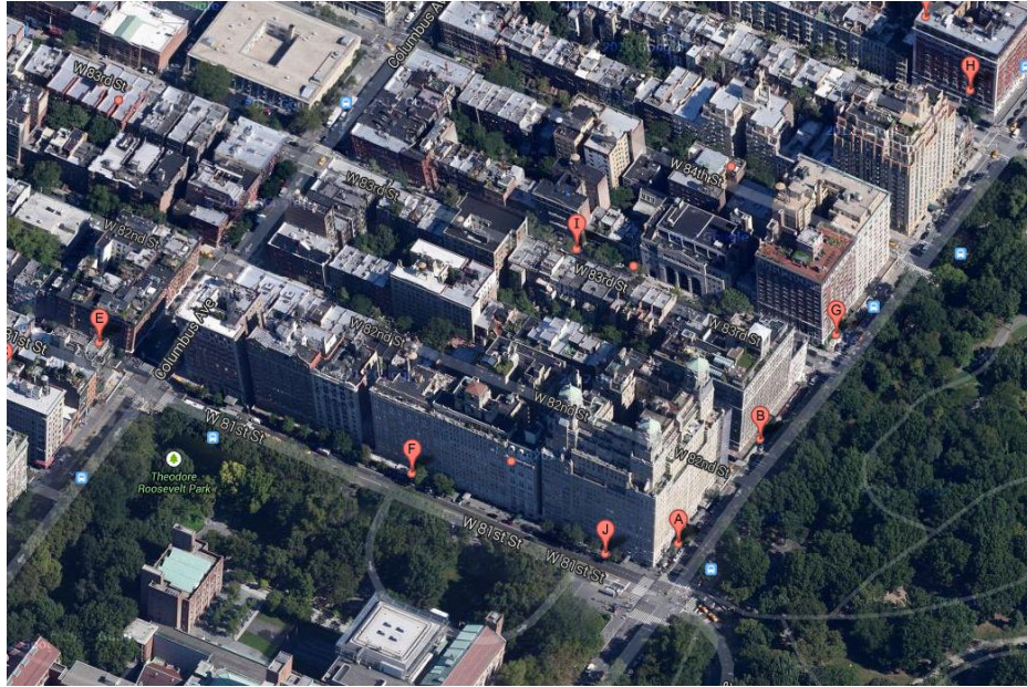
Figure 44. Aerial View of Amsterdam and 79 th Street
