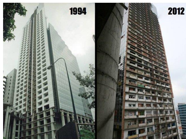
Figure 2. Tower of David 1994 and 2012
