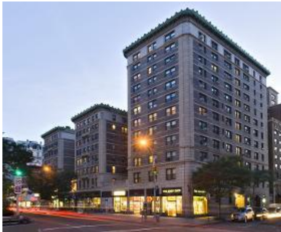
Figure 43. View of the Astor Building
